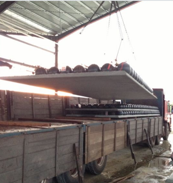
Loading BD precast elements onto the flatbed trailer
