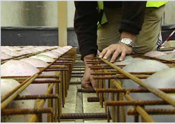
Sliding bottom splice bar central over joints
