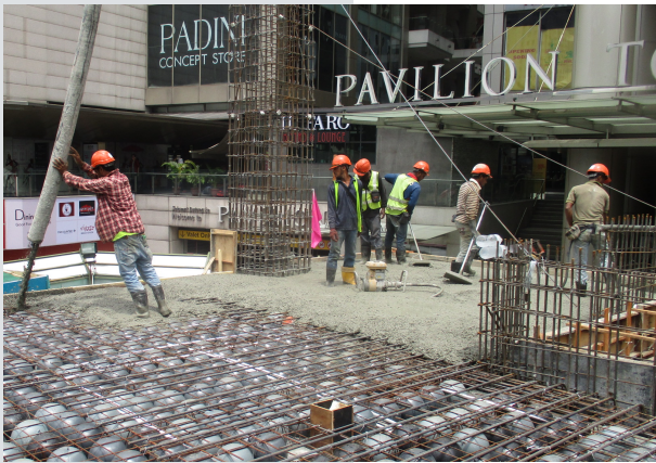
Pouring, Vibrating & Floating Site Concrete
