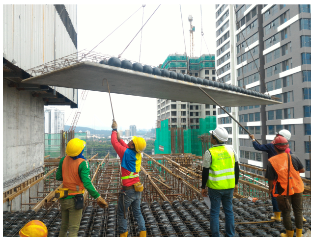
Lifting BD element onto position
