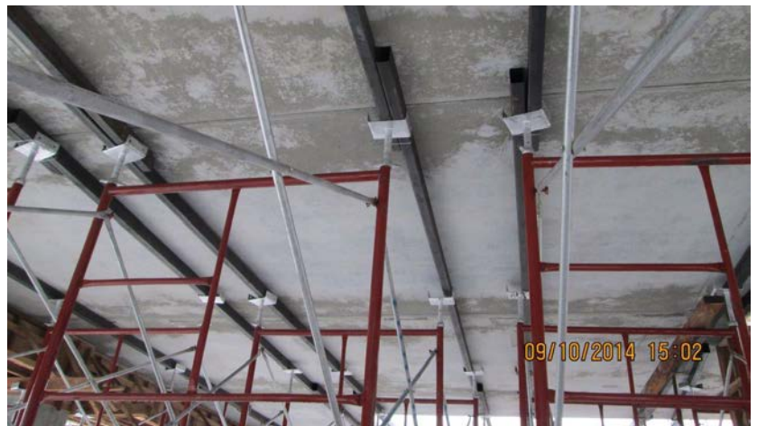
Typical arrangement of props and propping beams
